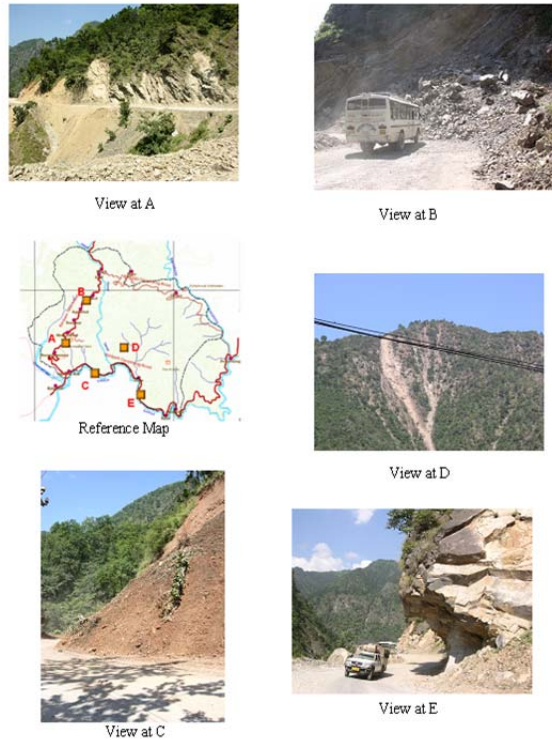
Fig. 5: View of landslides
